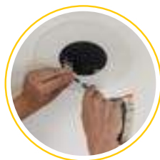
5. Electrical connection and installation of the new recessed ceiling light.
