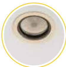
1. Old recessed ceiling light with larger ceiling cut-out.
